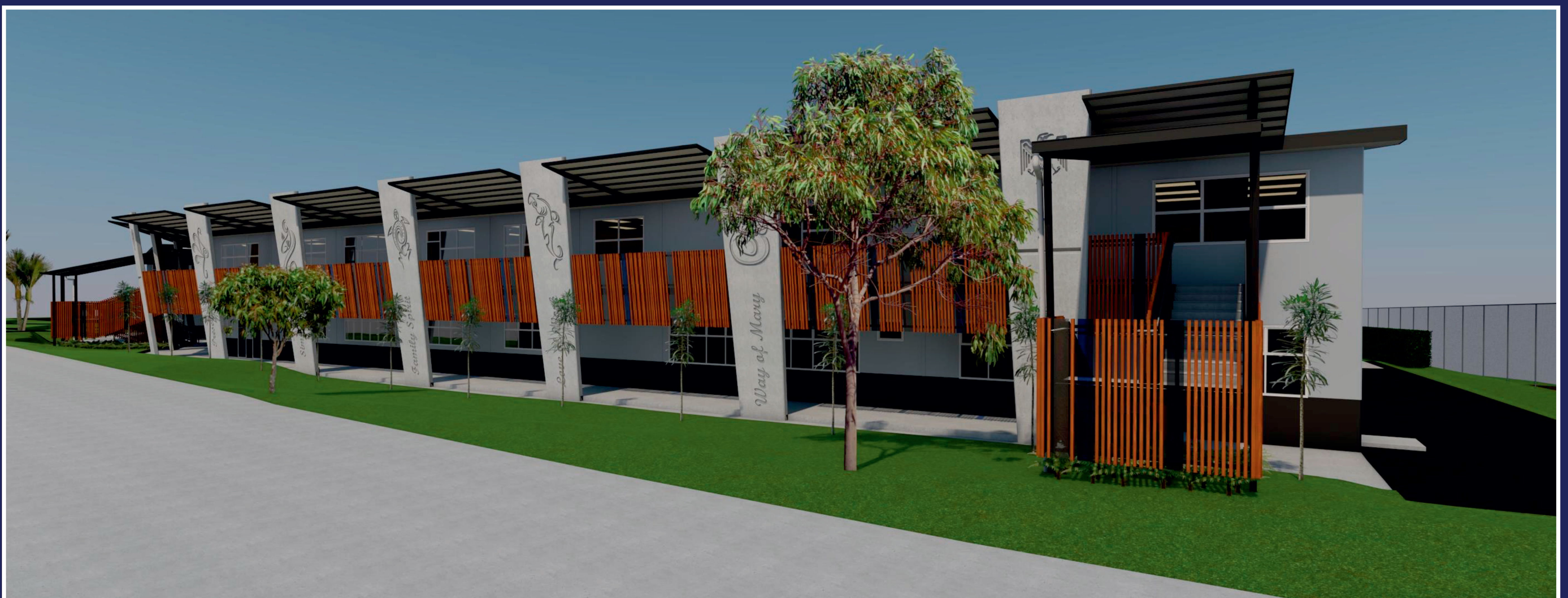
Striking street view, External walkways
